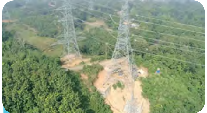
Two parallel transmission lines, converging in one line through a multi-circuit tower
